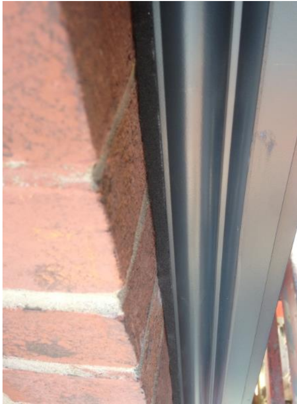
HANNOBAND BG1 application from the exterior (Hahne's Building, Newark, NJ)
