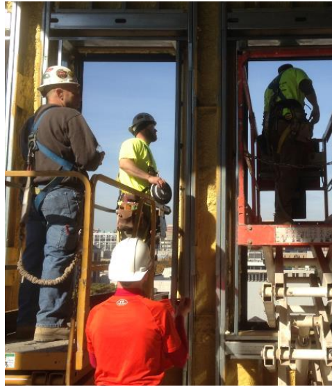
HANNOBAND BG1 application from the exterior (Hahne's Building, Newark, NJ)
