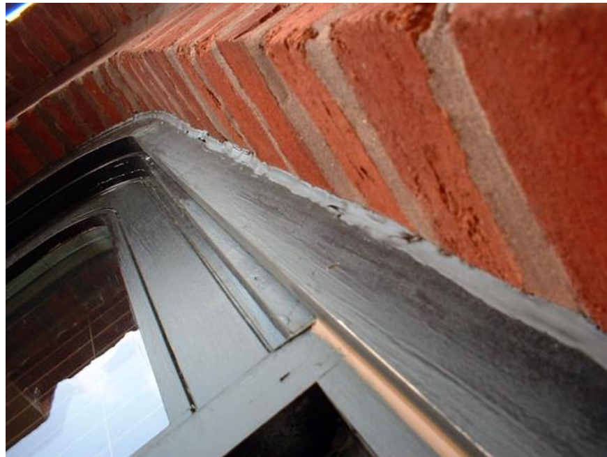
Typical US window installation – „Caulk & Walk“
