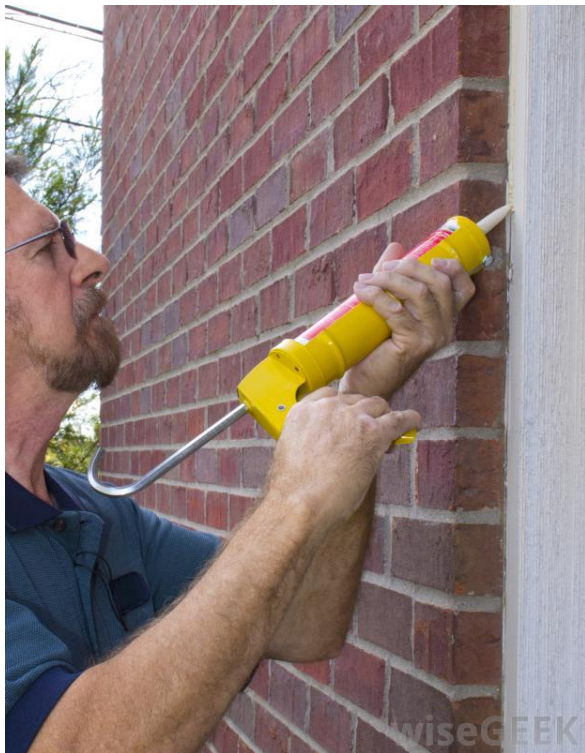
Typical US window installation – „Caulk & Walk“
