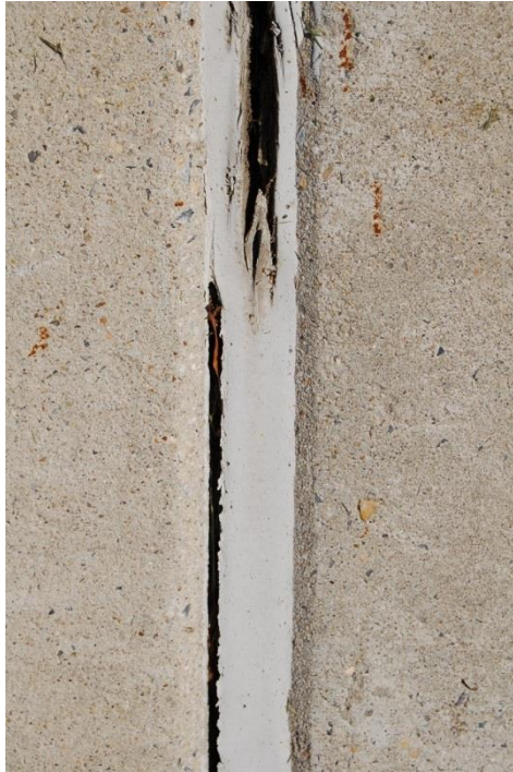
Water penetration from the exterior
